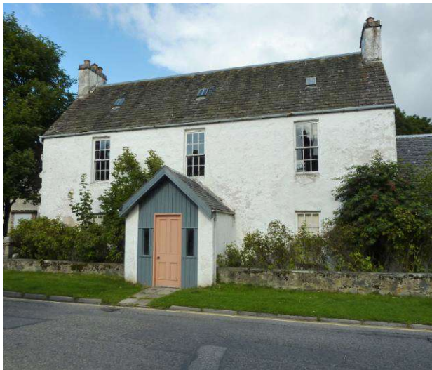
MacRobert House, Duke Street
